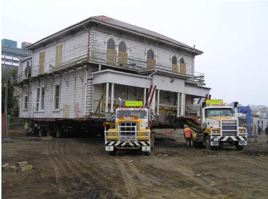
Figure 6: Floodplain building relocation in Illinois, USA (Source: [http://www.lakecountyil.gov/Stormwater/LakeCountyWatersheds/BMPs/PublishingImages/building\\_relocation.jpg](http://www.lakecountyil.gov/Stormwater/LakeCountyWatersheds/BMPs/PublishingImages/building_relocation.jpg)).
