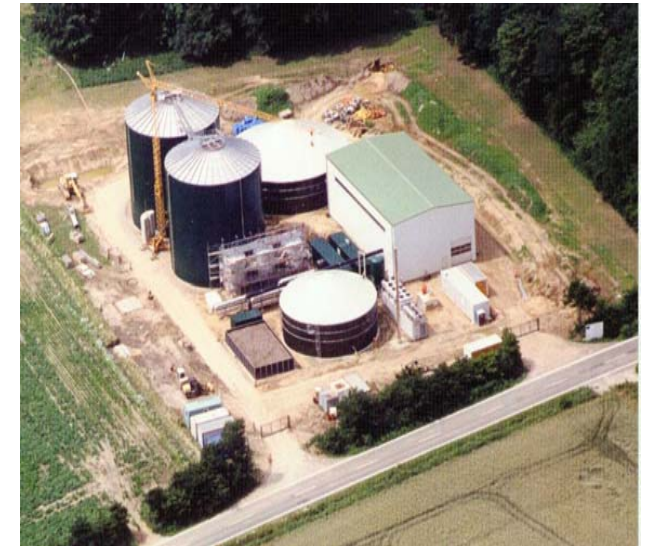
Biogasanlage in Albersdorf
